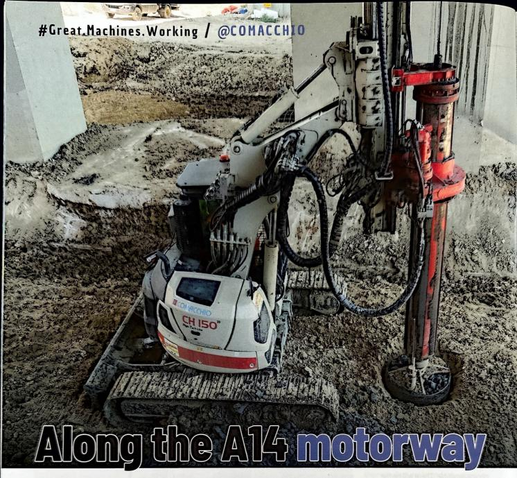
The project, which has a Comacchio CH 150 as its protagonist, involves the seismic retrofitting of a entire viaduct, and the simultaneous reinforcement of the foundations of all the piers and abutments
